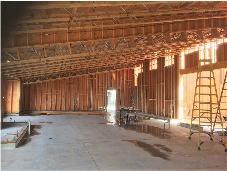
Classroom Interior View
